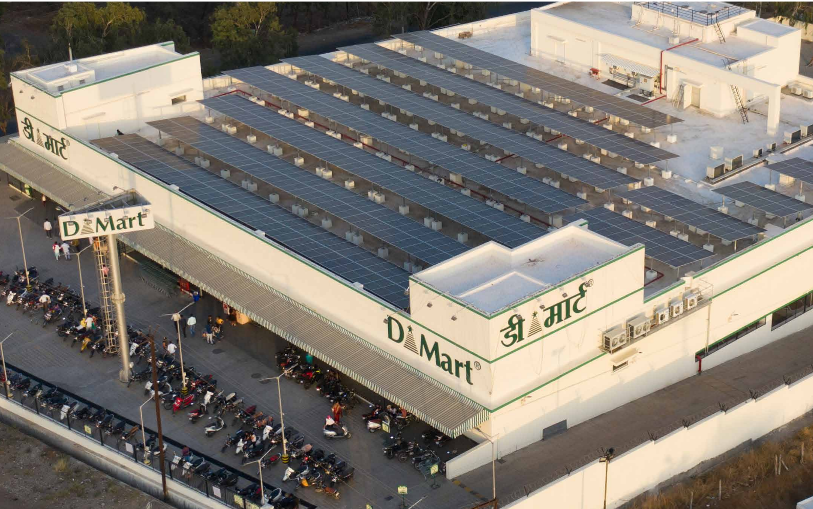
Rooftop Solar Panels
