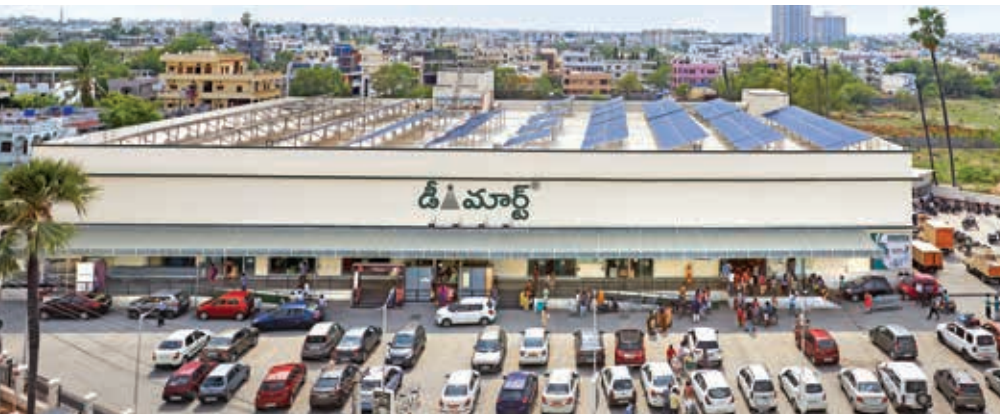
Rooftop Solar Panels
