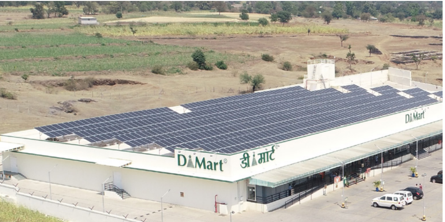
Rooftop Solar Panels
